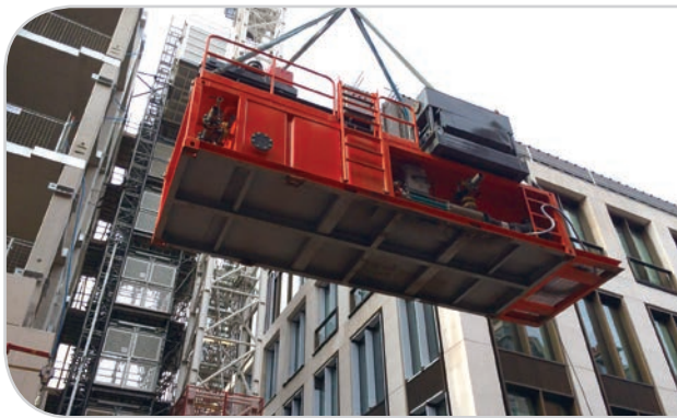
Geothermal Well Drilling Mud Cleaning
