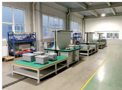
Electrical Control Equipment
