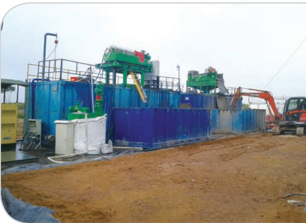
Inner Mongolia WBM Treating Project
