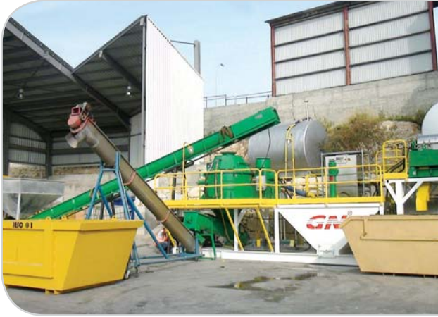
European Treating Plant Project
