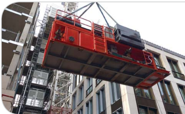
Geothermal Well Drilling Mud Cleaning
