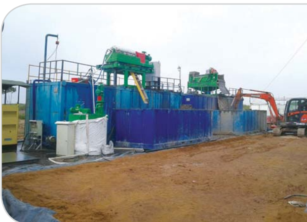
Inner Mongolia WBM Treating Project
